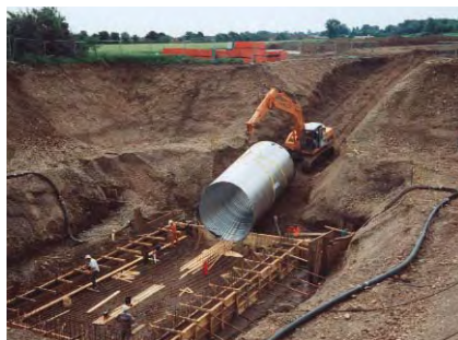
Construction of below ground crushing plant and conveyor tunnels at Catterick
