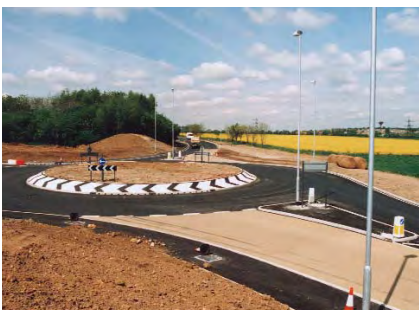
278 works South Elmsall
