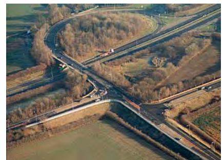
Welton Low Road junction improvements
