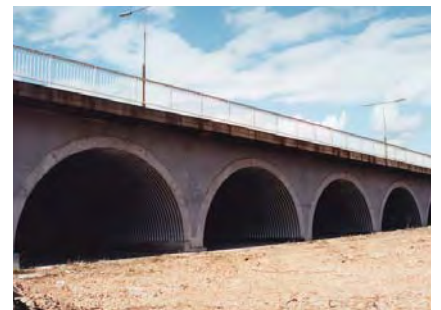
Design & build bridge strengthening Hessle Road flyover, Hull
