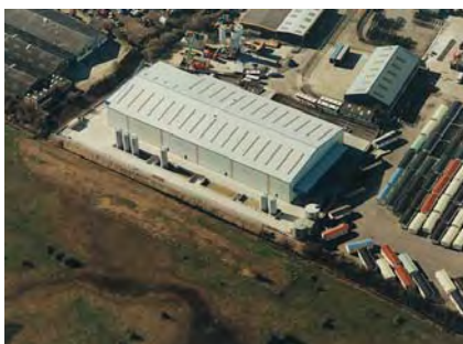
Design & build 58,000 sq. ft. factory, Beverley
