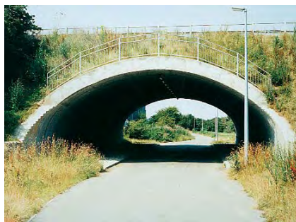
Design & build bridge strengthening, Marfleet Lane, Hull
