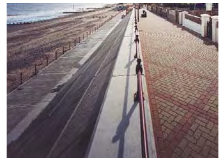
Reinforced concrete sea defence works, Withernsea
