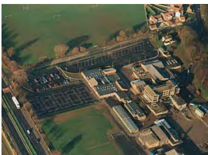
Provision of new car park & tennis courts, South Hunsley School, North Ferriby
