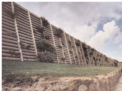
Cliff stabilisation Scarborough
