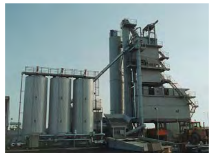
Design & build reinforced concrete works for new asphalt plant at Shoreham
