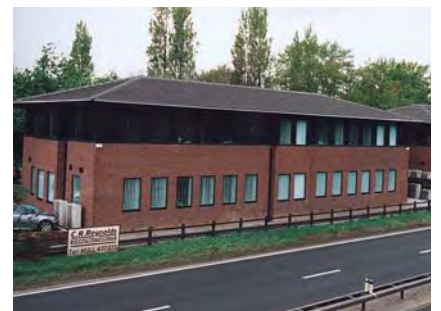
Design & build two office blocks, Hessle
