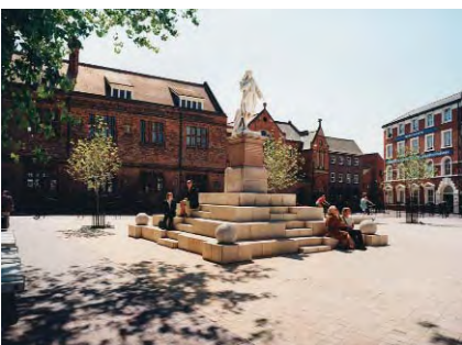
Repaving works, Market Place Hull
